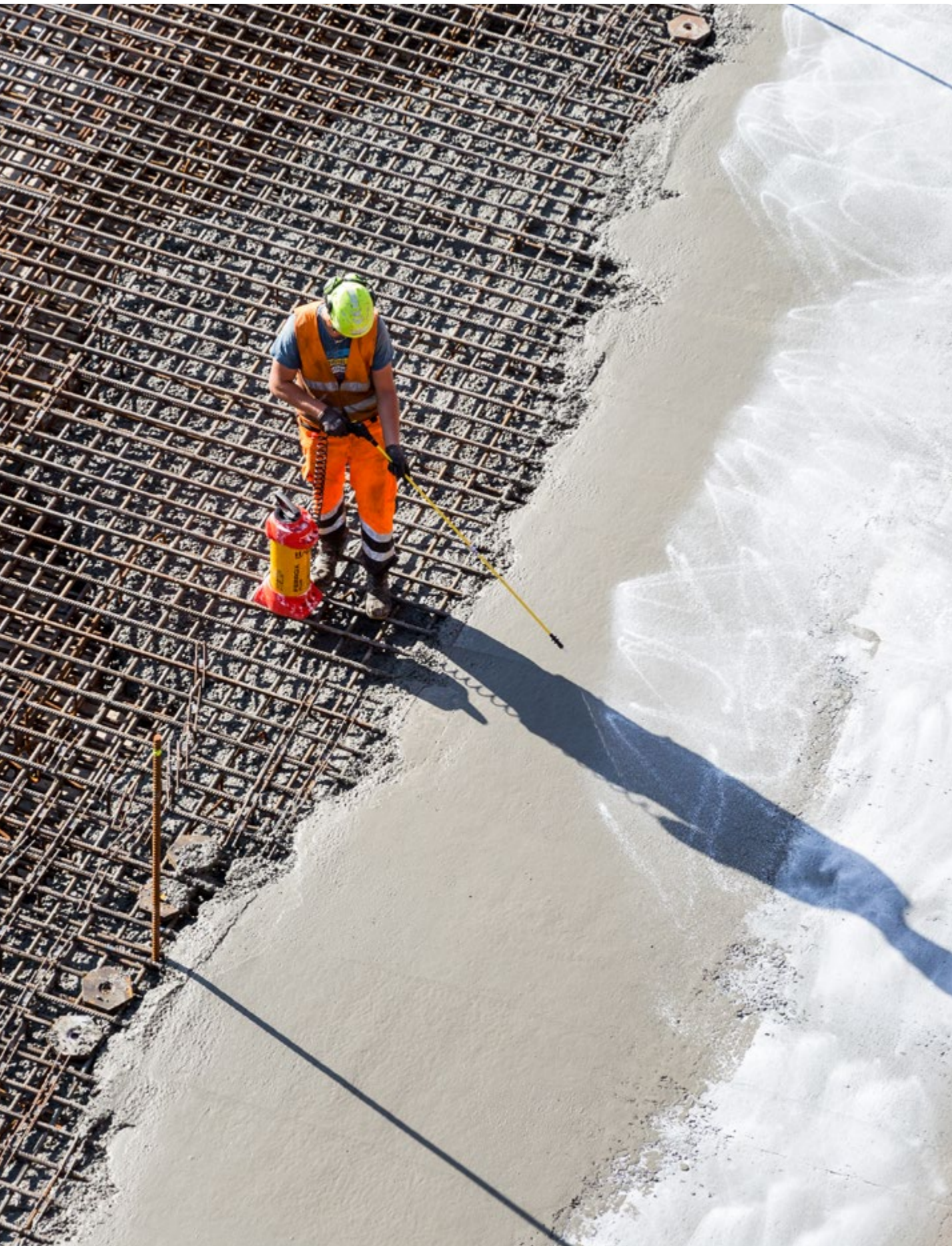
Concrete casting at PensionDanmark's construction project at Kronløbsøen
